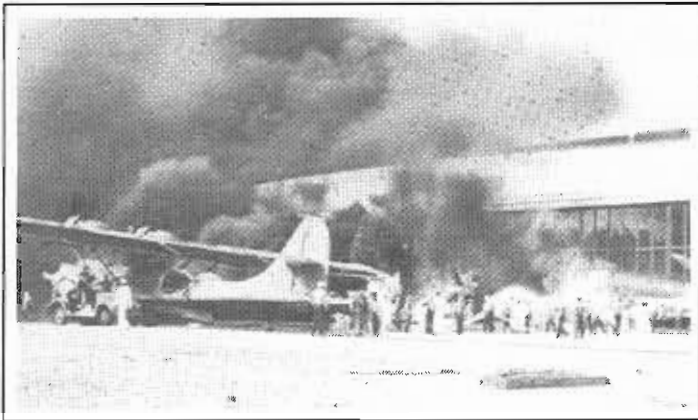
FORD ISLAND took some very big hits. Most of the aircraft and other equipment was destroyed. Here, firefighters do their best to save several PBV's. The Japs did a very thorough job.
